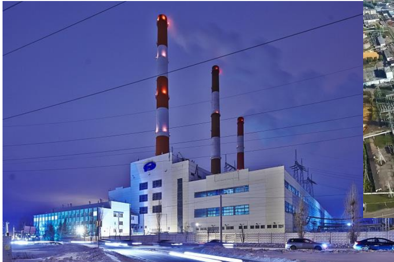
Ufa power station
